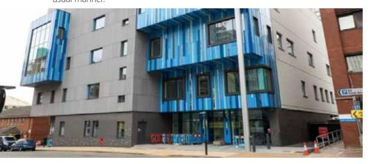
The 7,765m² ffacility situated on a tight city centre corner site meant that space for storage and deliveries was at a premium. The team therefore adopted modern methods of construction (MMC). Through prefabrication and modularization, disruption and site congestion were minimized improving installation efficiency which was reflected in the overall construction programme.
